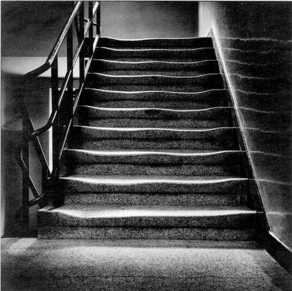
[Image: Simon Norfolk . Staircase at Auschwitz, with worn footsteps.]
